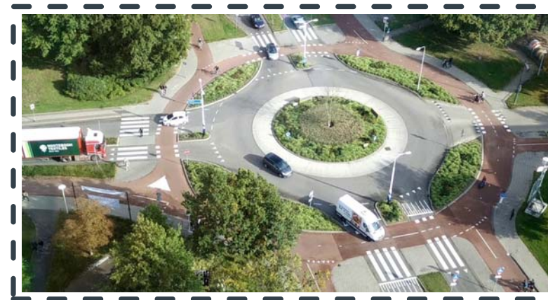
Bike/Pedestrian Facilities in Roundabout
