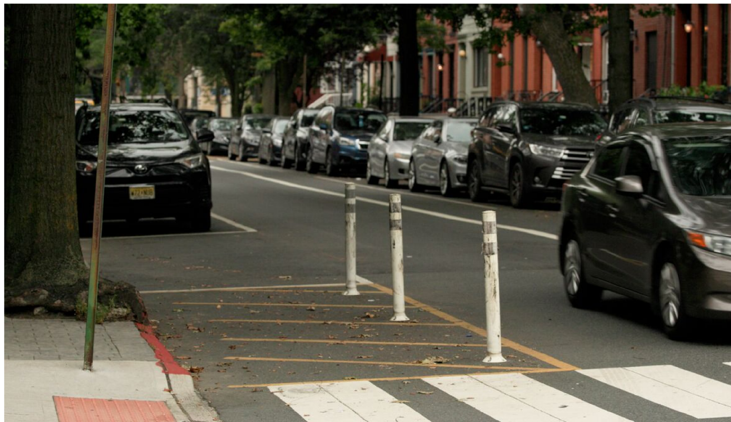
Plastic flexposts keep vehicles away from an intersection in Hoboken. Photo: Bloomberg News
