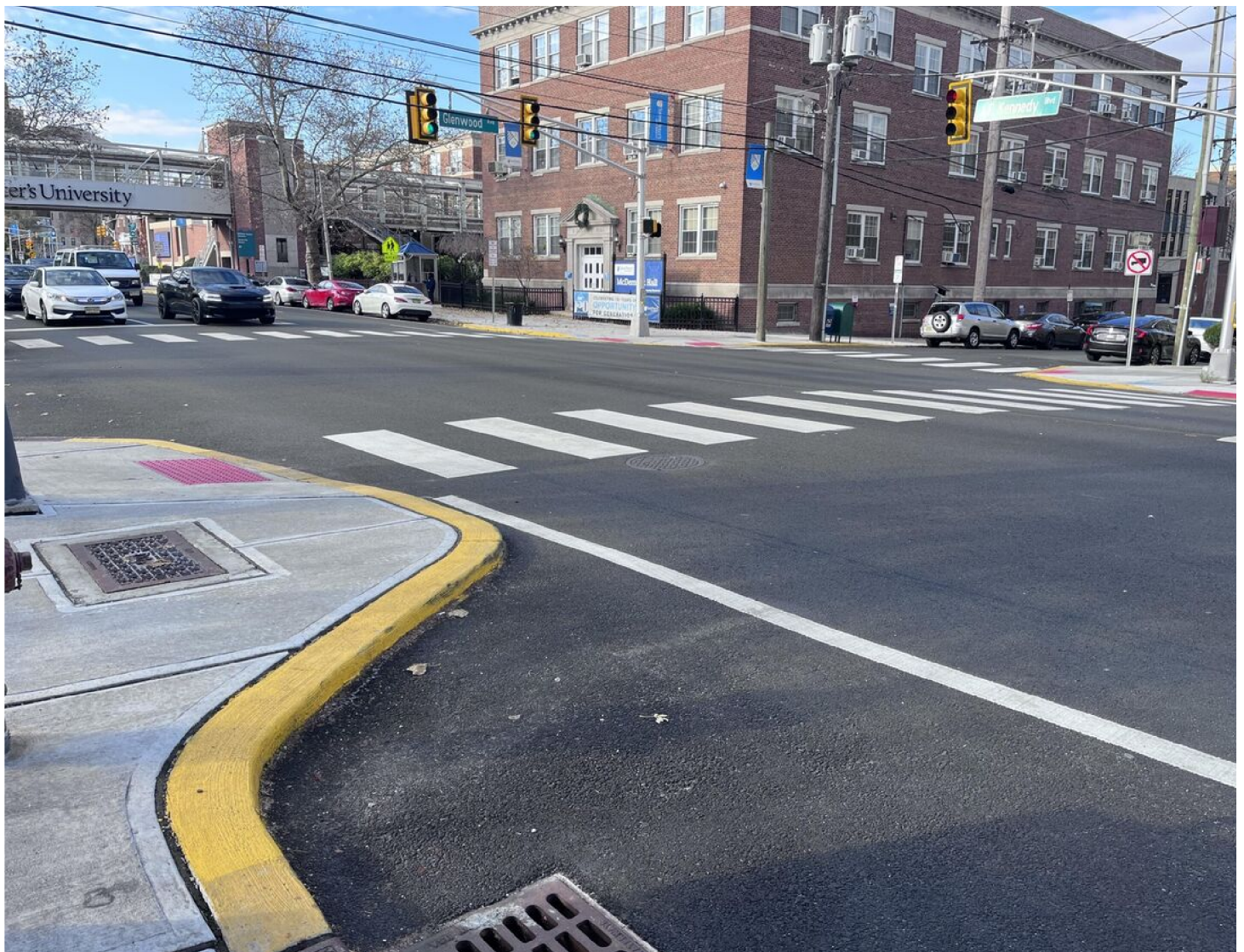
Paved curb extensions in Jersey City have been installed as part of that city's traffic safety makeover. Photos: John Surico/Bloomberg CityLab
