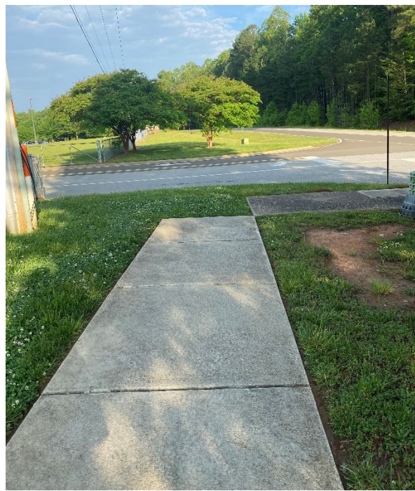
End of sidewalk at the eastern driveway
