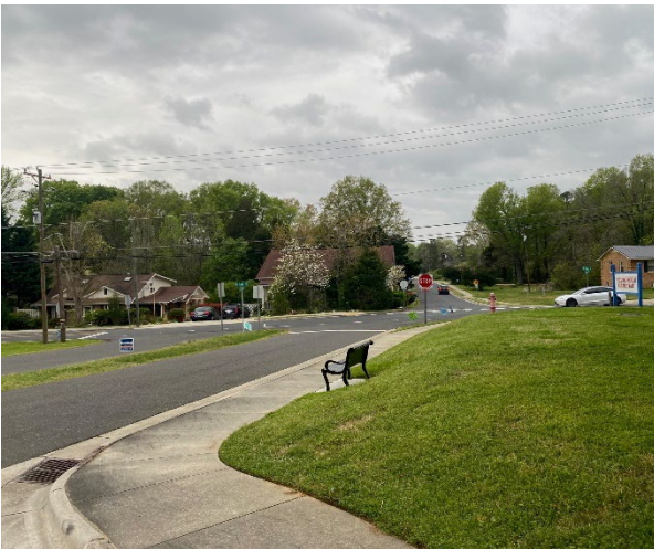
Standing on W Union Street looking west at the skewed intersection with N Nash Street and Hayes Street.
