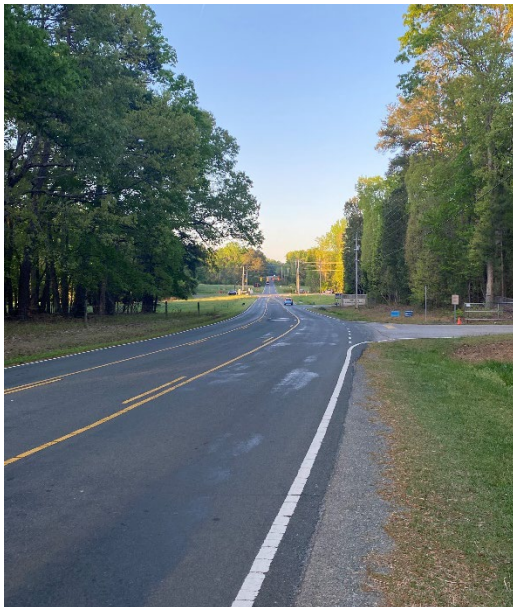
Looking southwest down New Hope Church Road towards the intersection with NC 86
