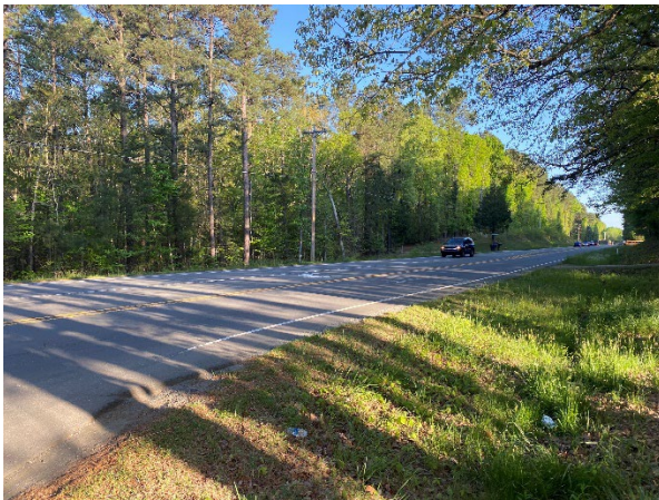
NC 86 left-turn lane onto Benton Drive
