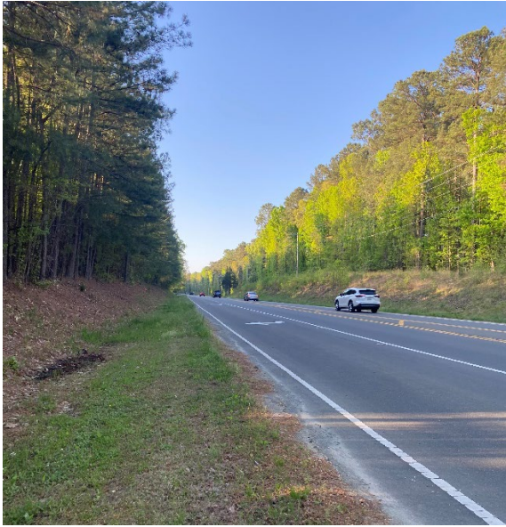
NC 86 right-turn lane onto Benton Drive
