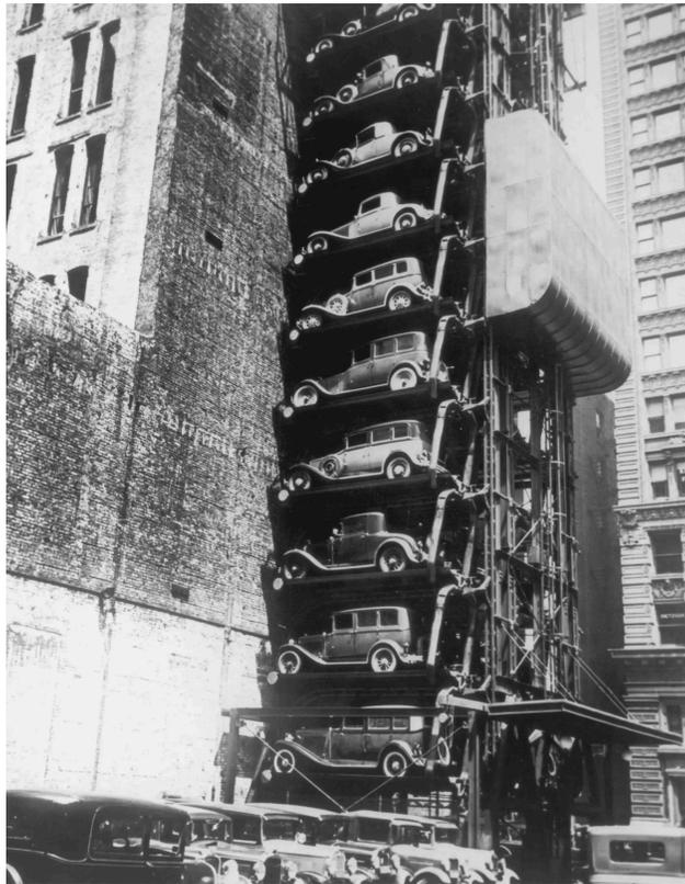
The “vertical parking machine” of 1932 could hold 48 cars.
