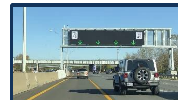
5. Hard Shoulder Running
