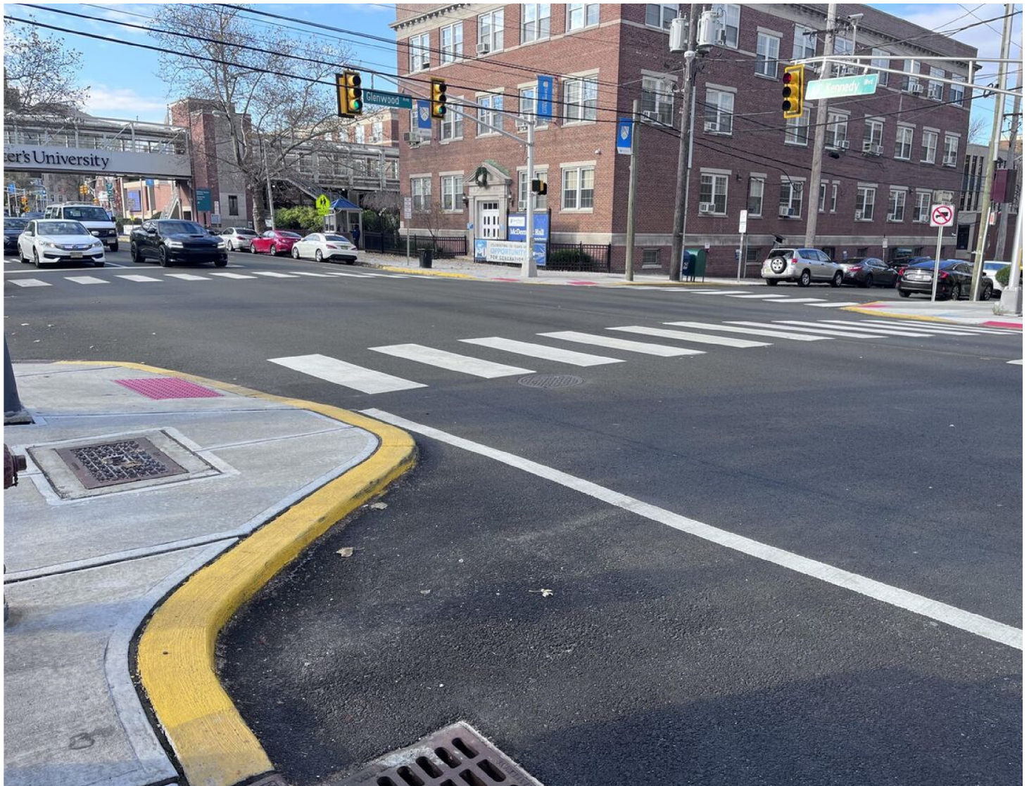
Paved curb extensions in Jersey City have been installed as part of that city's traffic safety makeover. Photos: John Surico/Bloomberg CityLab
