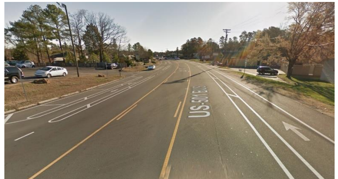
Figure 18: Segment 4 – Chapel Hill Road to University Drive
