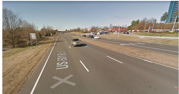
Figure 17: Segment 3 - US 15-501 near Tower Road
