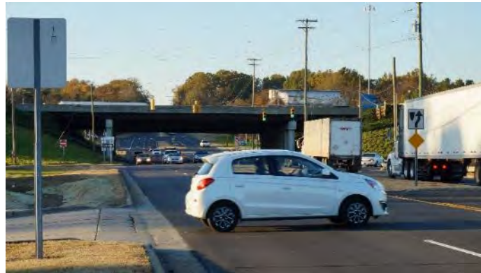
Looking west towards I-40/I-85
