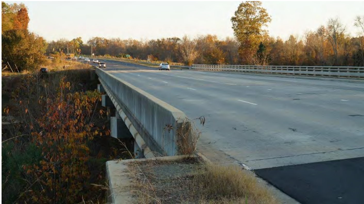
Looking east across Haw River Bridge
