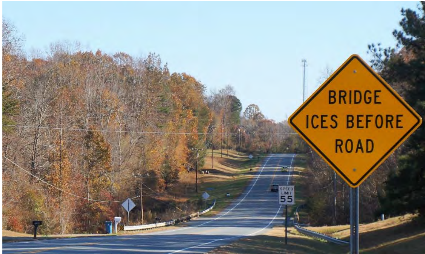
Looking east at Haw Creek Bridge
