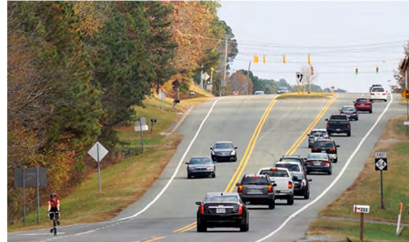
Roadway shoulder west of Carrboro
