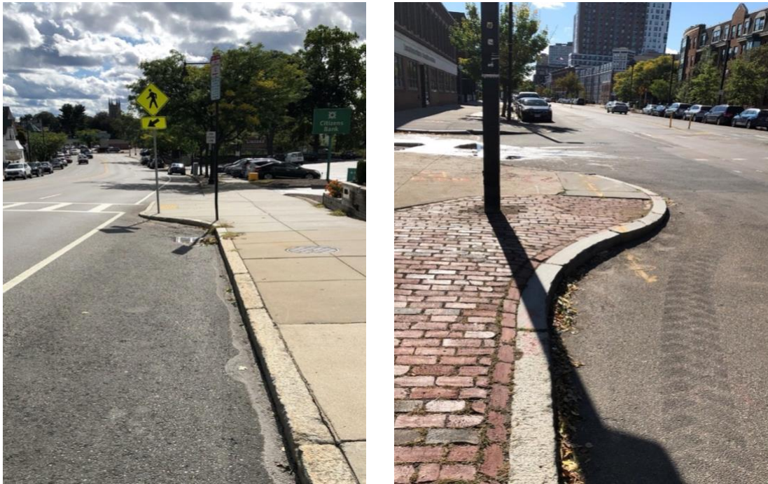
Curb extensions crossing Centre Street (left) and Tremont Street (right) in Boston, Massachusetts.
