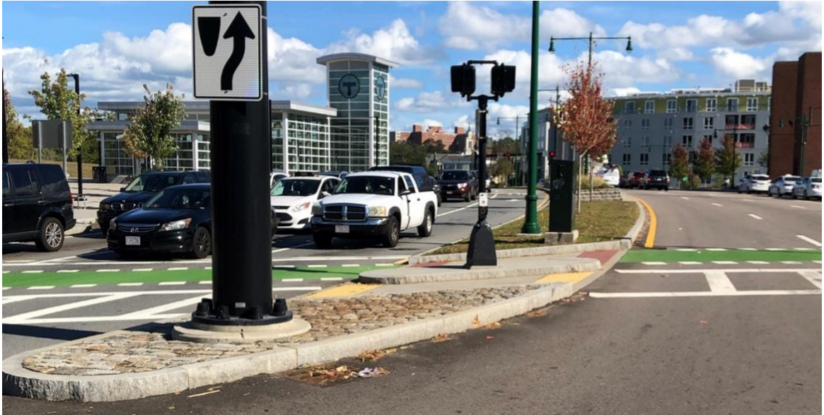
Pedestrian crossing island on the Arborway at Forest Hills looking east from the intersection with South Street in Boston, Massachusetts.
