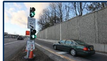
B. Ramp Metering
