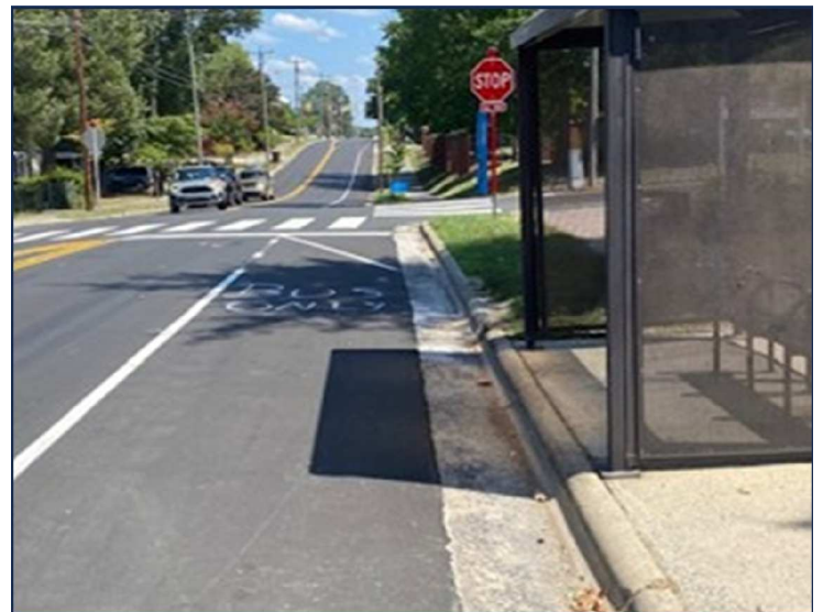
Four-way stop at Lawson Street and Concord Street. Intersection is now safe for pedestrians and students.
