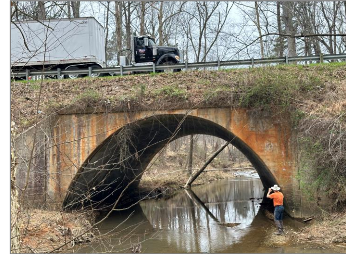
US 70 culvert over Stony Creek in Orange County
