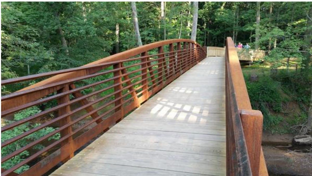
New footbridge linking Hillsborough's Riverwalk with historic speedway trail.
